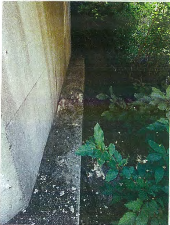
Photo 25 – View of North Abutment
