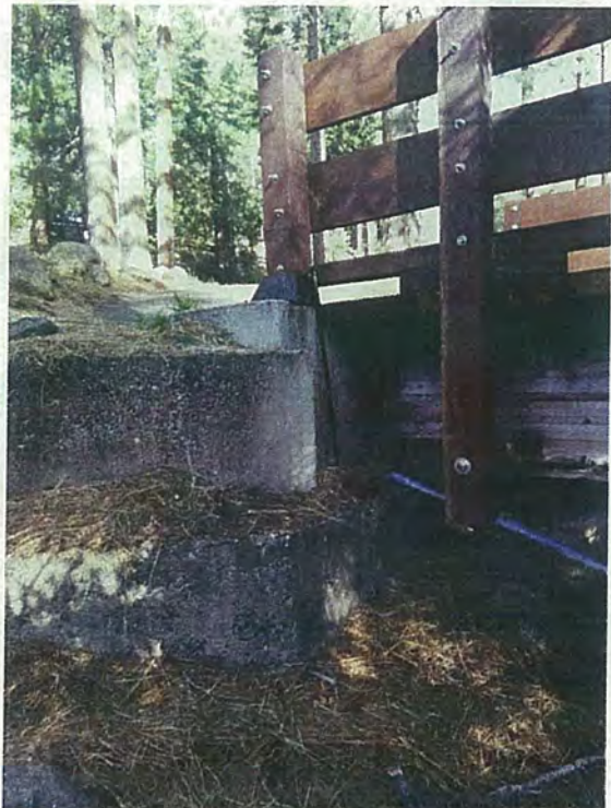
Photo 16 – View of West Abutment
