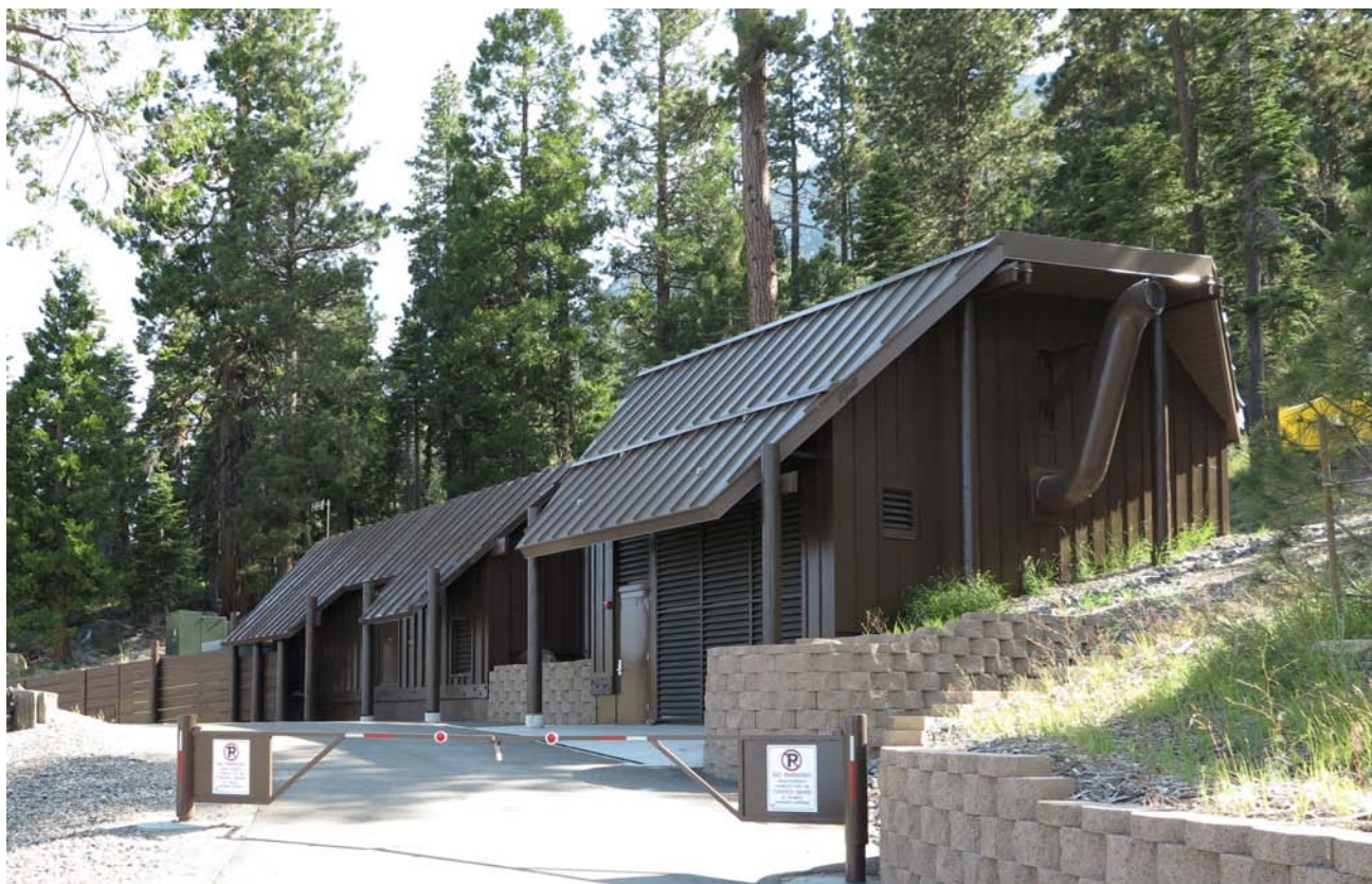
Spooner Pumping Station
