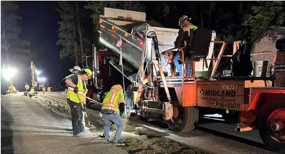
Overall, the conditions were challenging following the heavy winter as the crew battled high groundwater levels and leaking stormwater pipes in the trench. Large boulders and bedrock were encountered – as is typical in the Tahoe area – and required specialized crews and equipment to safely remove them
