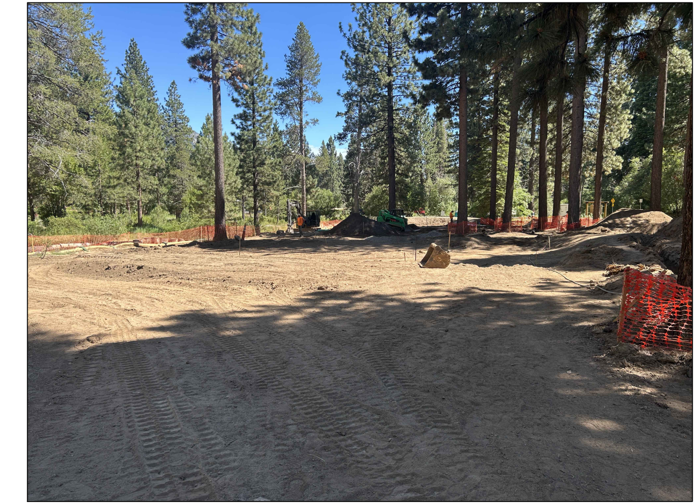
JULY 6: SITE CLEARED AND GRUBBED
