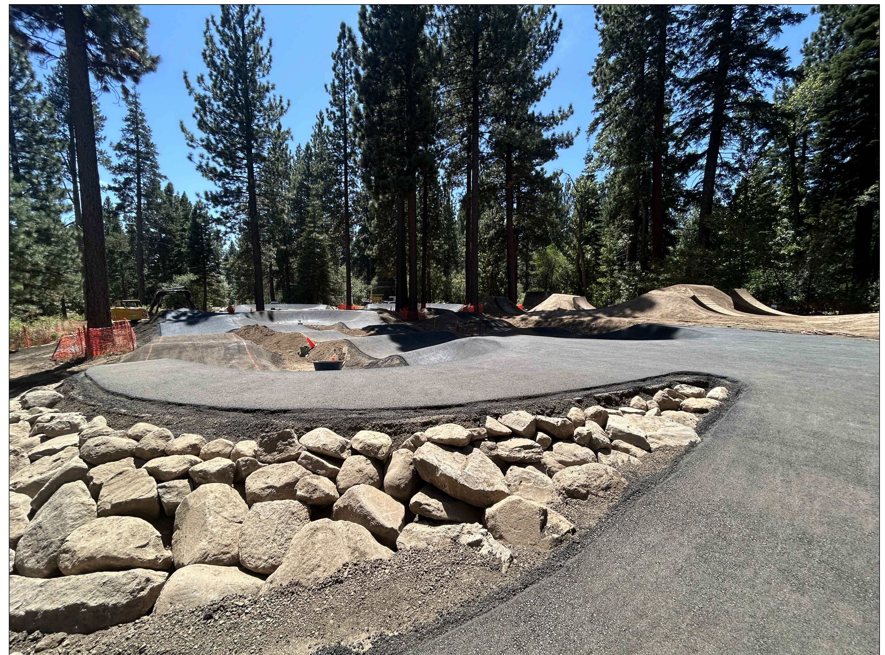
AUGUST 14: PAVING NEARLY COMPLETE
