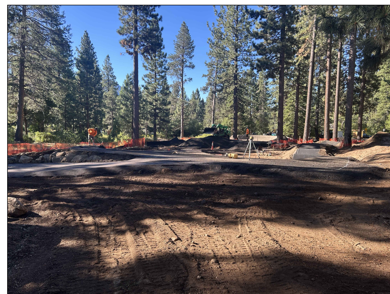
JULY 28: PAVING AND SHAPING IN PROGRESS
