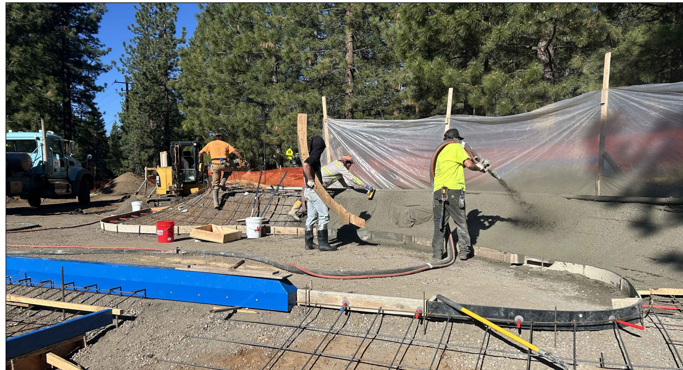
OVER 150 CUBIC YARDS OF CONCRETE AND SHOTCRETE USED
