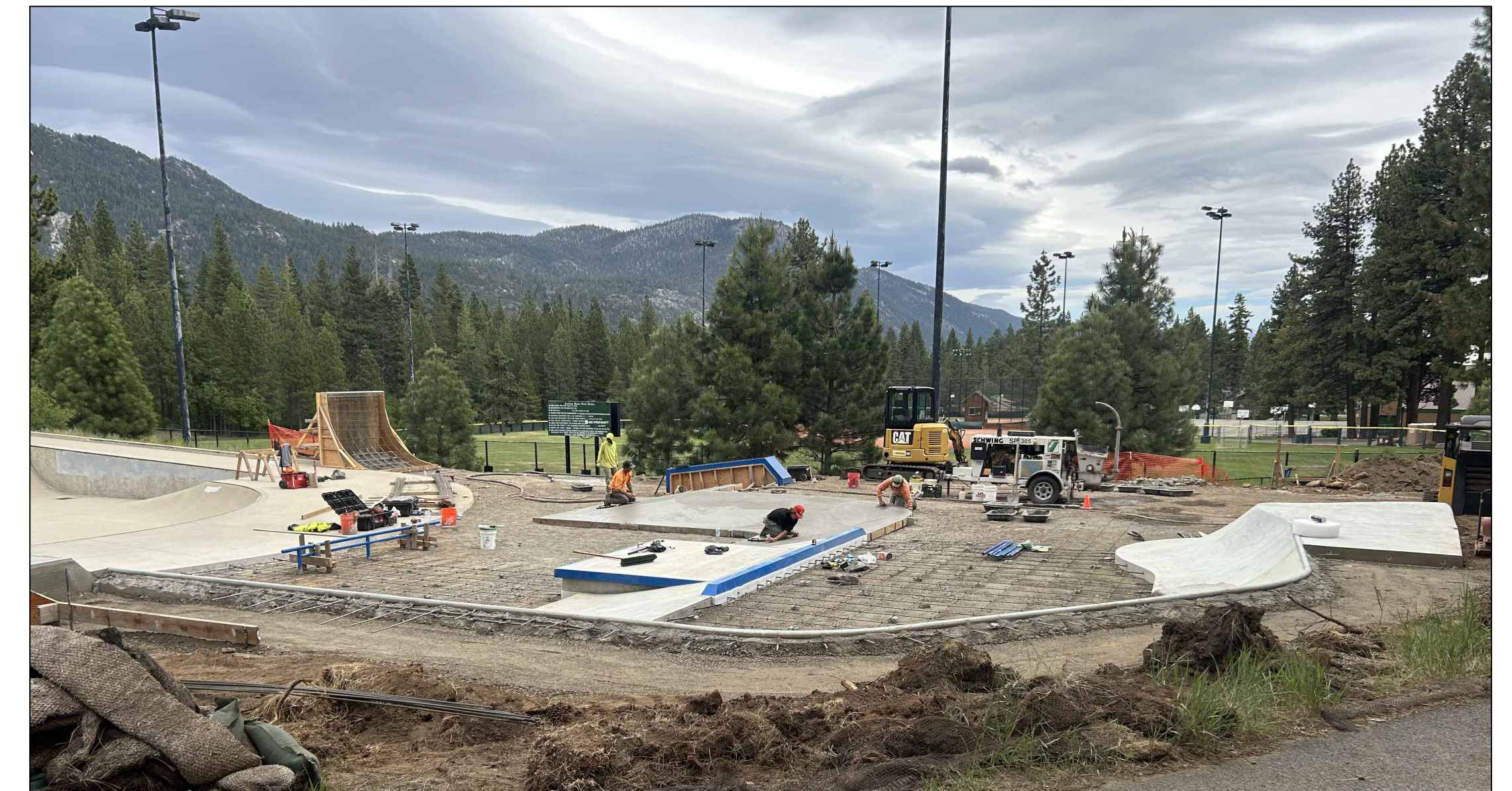
NEARLY 3000 POUNDS OF REBAR INSTALLED
